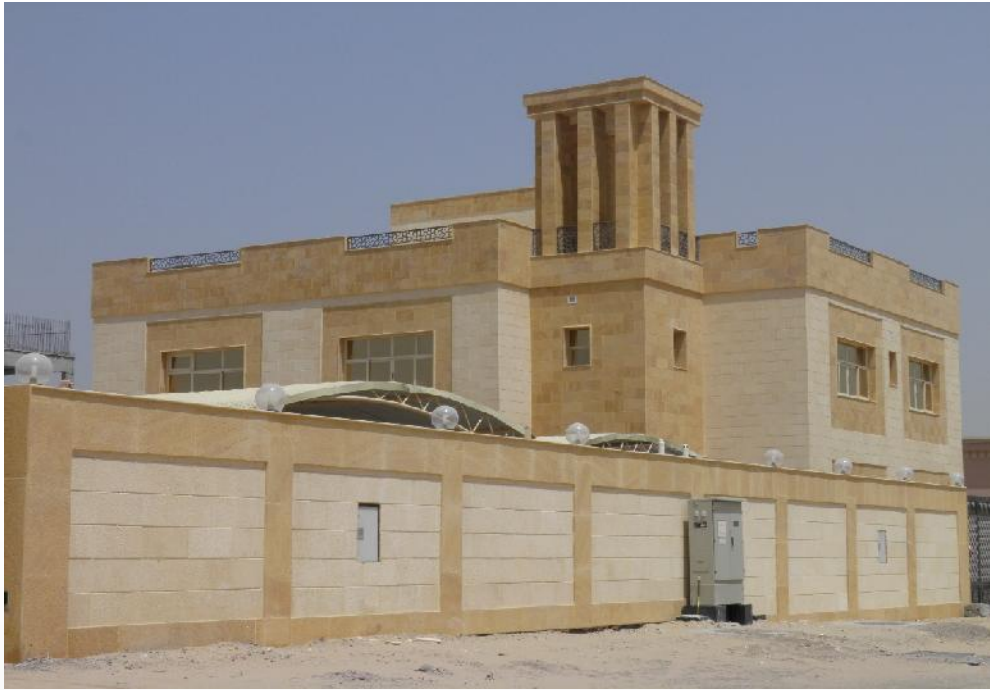
Project :(Villa Two Private) for Mr.Mohammed Essa Bin Qeba Location : Al Barsha South
