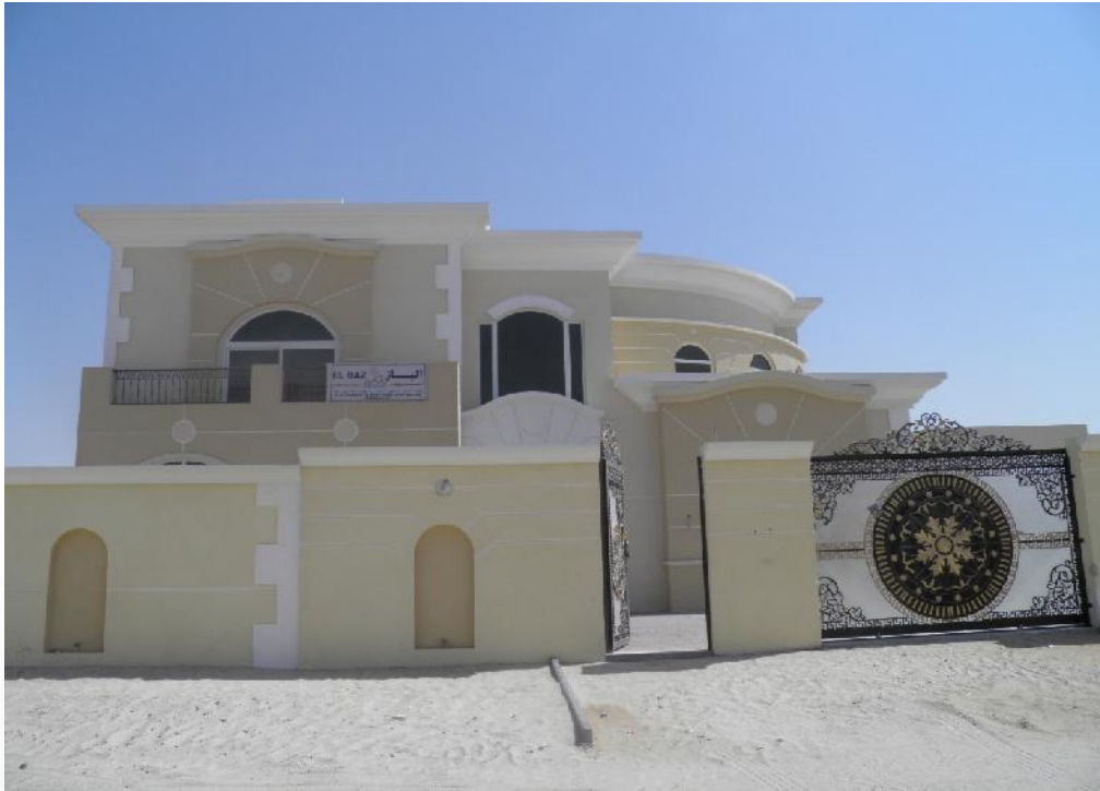
Project :(Private Villa G+1 ) for Mr. Jassem Slaman Mohamed Location : Al Barsha South First
